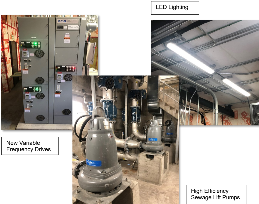
Figure 2.4 Upgrades to Harbour Street Lift Station
