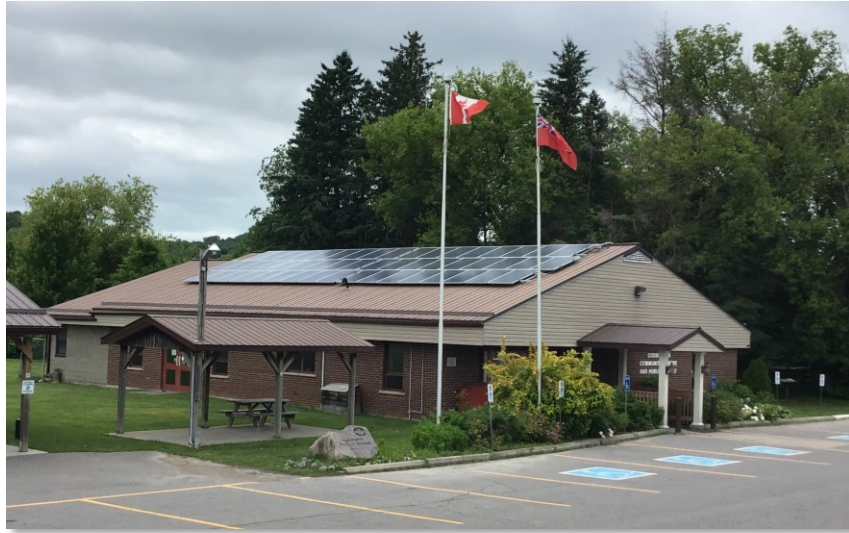
Figure 1.1 Solar Panels - Codrington Community Centre
