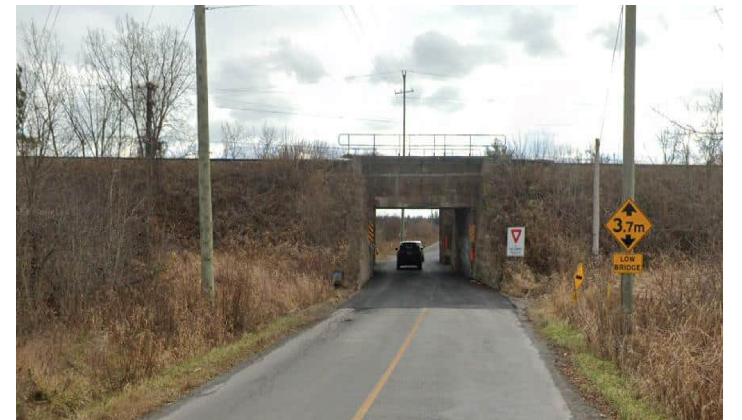
Boes Road Underpass (Looking South)
