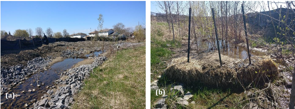
Figure 14. Rip-Rap Channel (a) and Sediment Accumulation Behind Check Dam (b) in Arena Creek North Tributary
