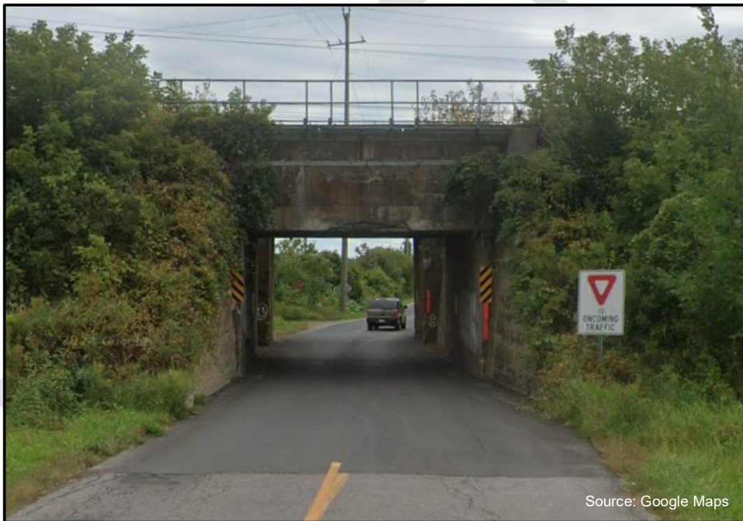
Exhibit 2.9 Boes Road Rail Underpass
