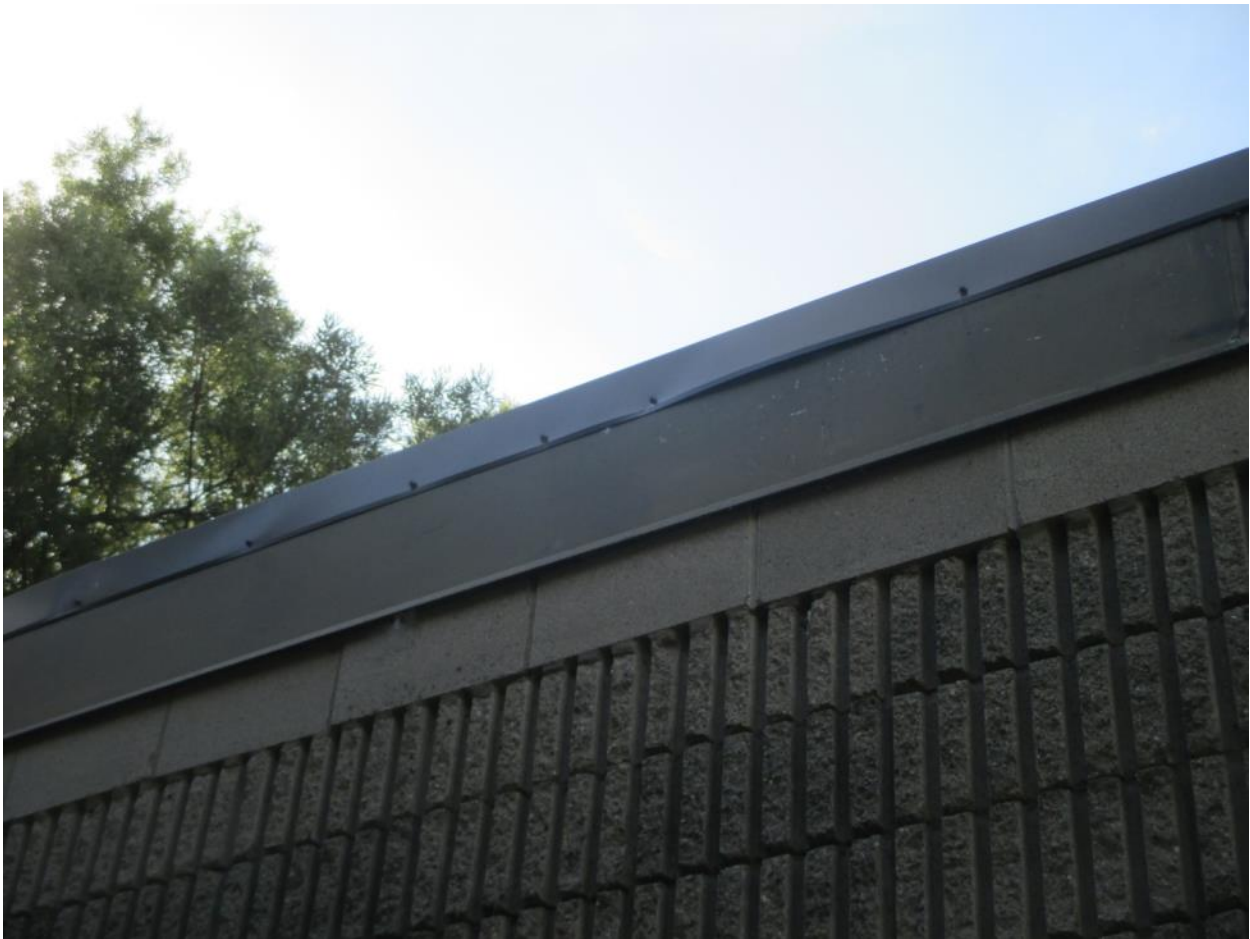
ID01_AS10: Perimeter Drip Edges
