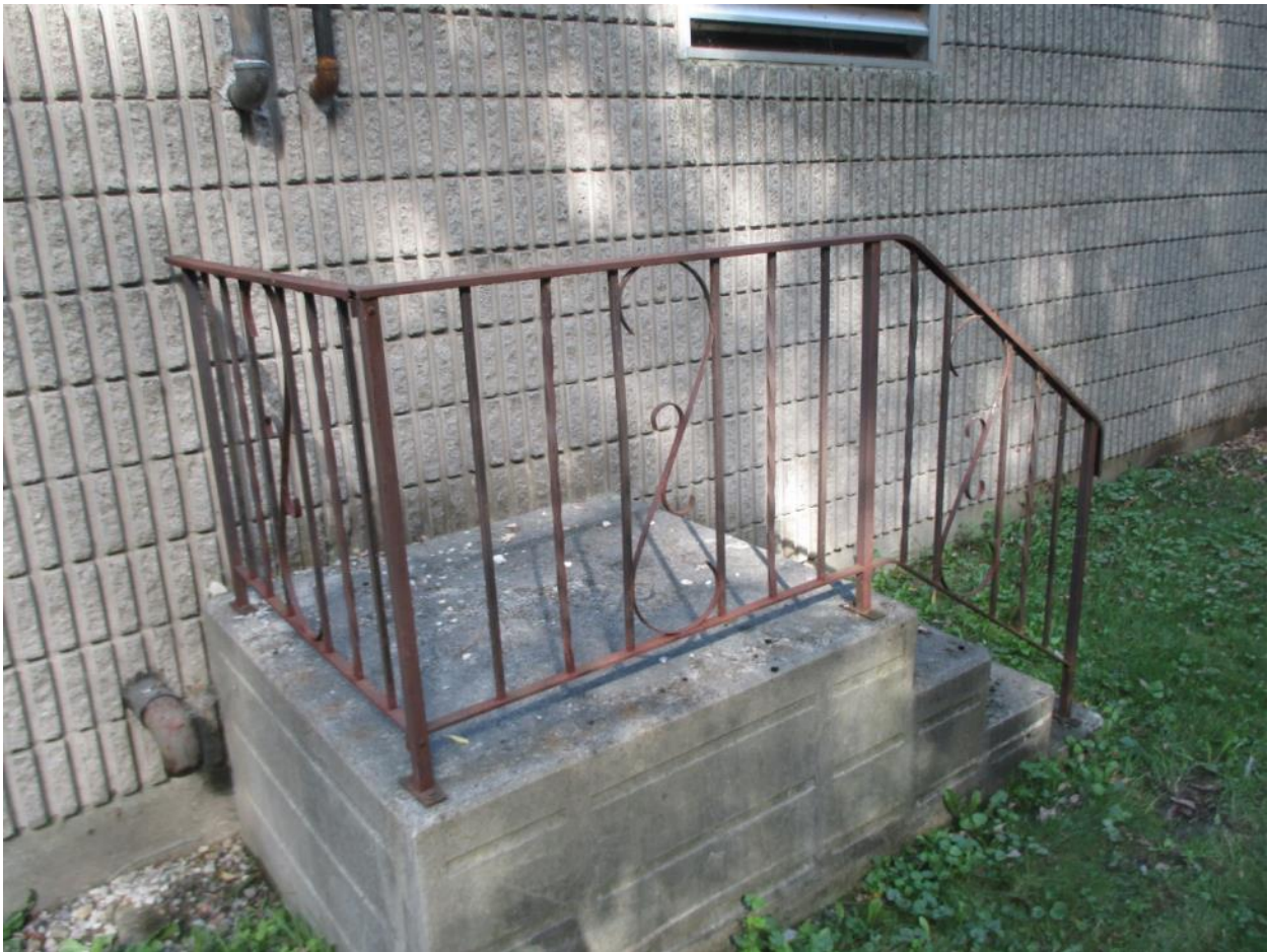
ID01_AS13: Ferrous Handrail
