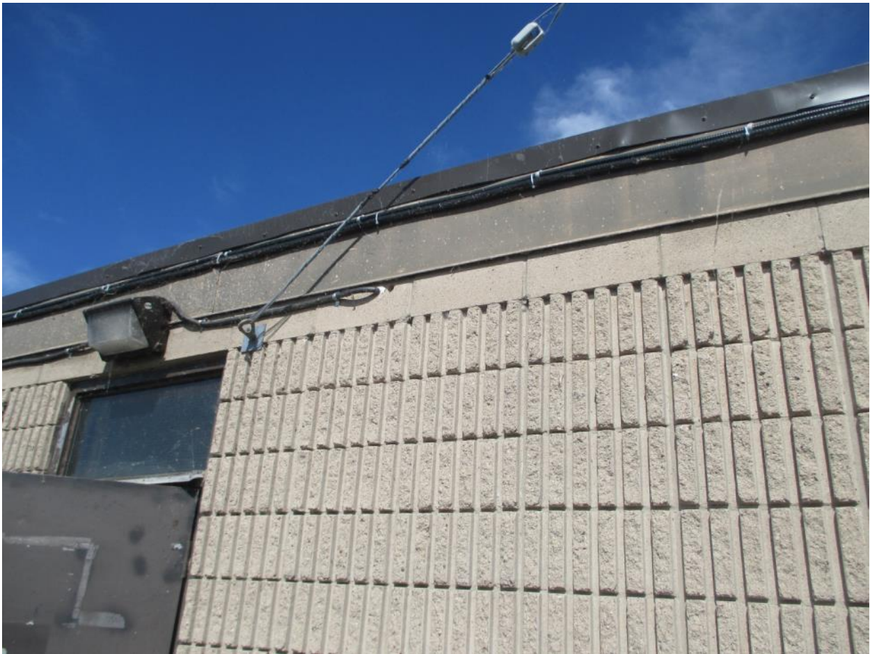
ID02_AS05: Perimeter Drip Edges
