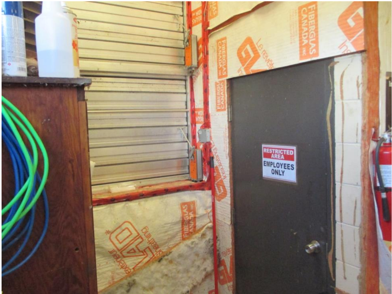
ID01_AS08: Insulation Covering Concrete Superstructure
