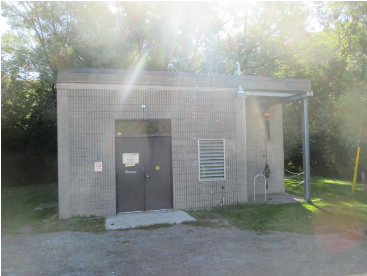
ID01_AS01: Sewage Pumping Station Located at Grade
