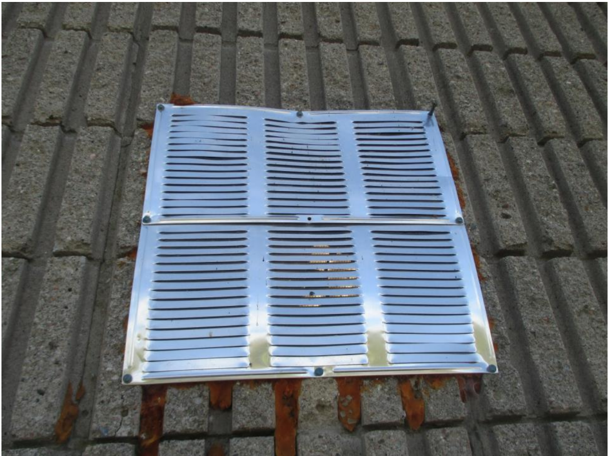
ID02_AS07: Potential Pathway for Water and Insects
