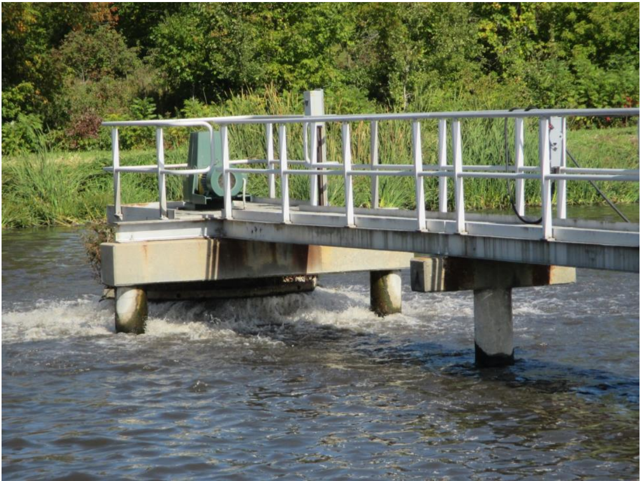
ID02_AS13: Aluminum Walkway
