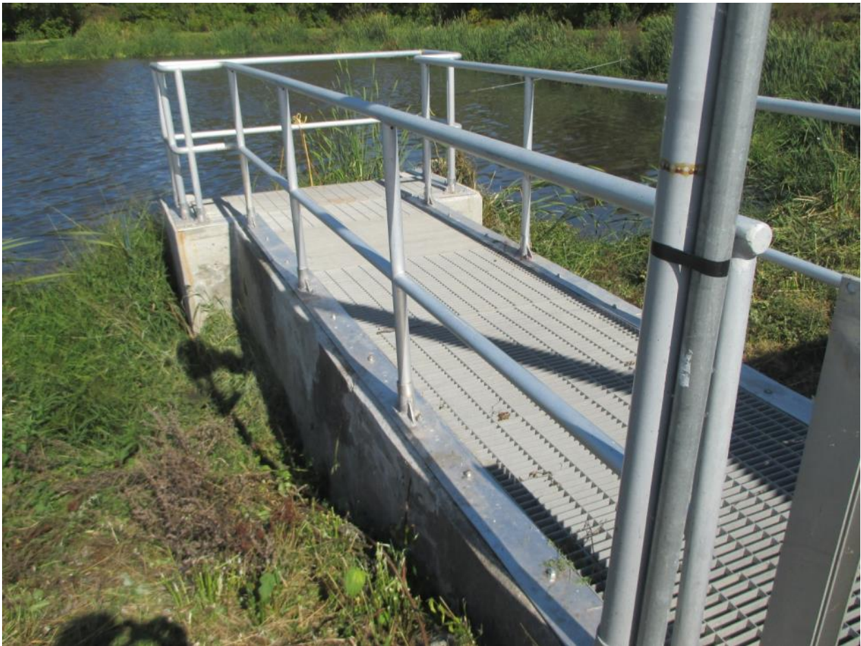
ID02_AS12: Recently Upgraded Cast in Railings
