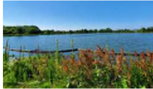
Lagoon Treatment (feasible for mechanical plant converted from lagoons; modifications option available)
