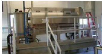
Rotary Drum Thickener (requires sludge storage)
