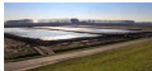
Sludge Drying Bed/ Storage Lagoon
